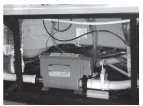
After the spa has been placed on an approved surface and has been correctly wired by a licensed electrician, inspect all plumbing connections in the equipment area of your spa. Ensure that these connections are secure and that they did not loosen during shipment.
